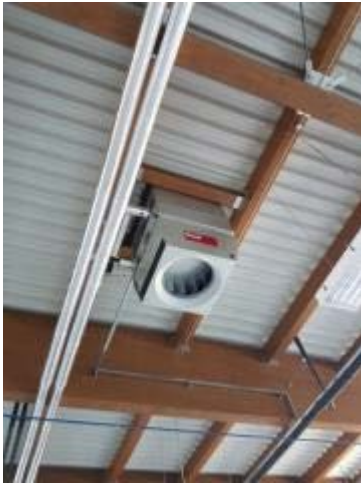
Figure 12: TopVent DHV unit inside the hall (source: Pannonian wood competence centre gallery)
