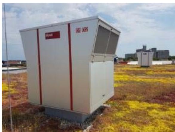
Figure 11: RoofVent RH units on the green roof (source: Pannonian wood competence centre gallery)
